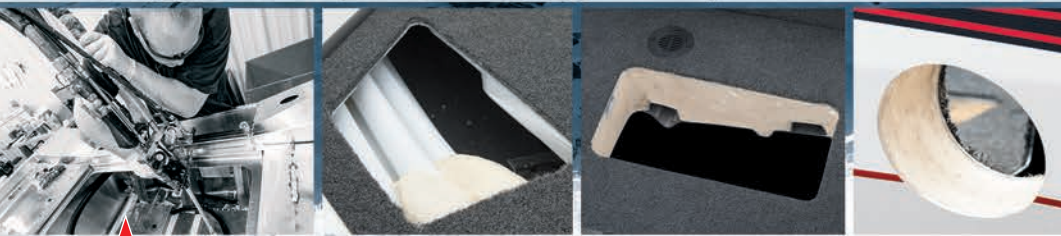
Injecting foam into inner cavities
